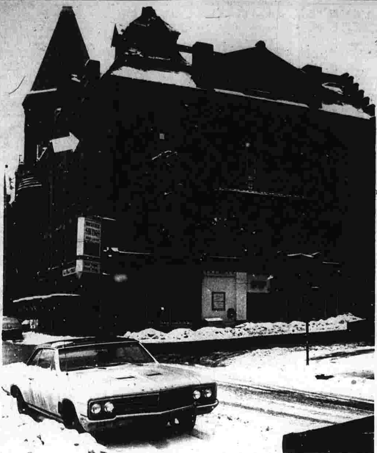
Henry Building at corner of Park Pl. and Park St. in Rockville. Arrow points to weakened wall.
